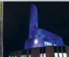
Northern Lights Cathedral, Alta, Norway / Schmidt Hammer Lassen Architects & Kolbjörn Jenssen
