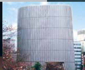
Showa Hall, Tokyo, Japan / Kikutake Architects
